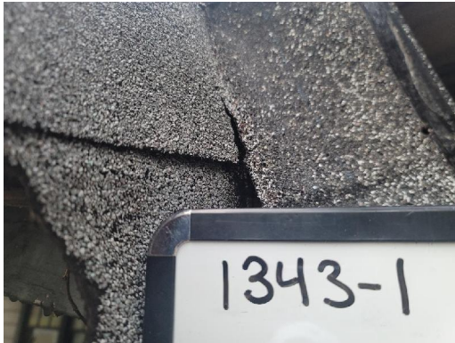
1343-1 Asphalt Shingle/Tar Typical Exterior Roof
