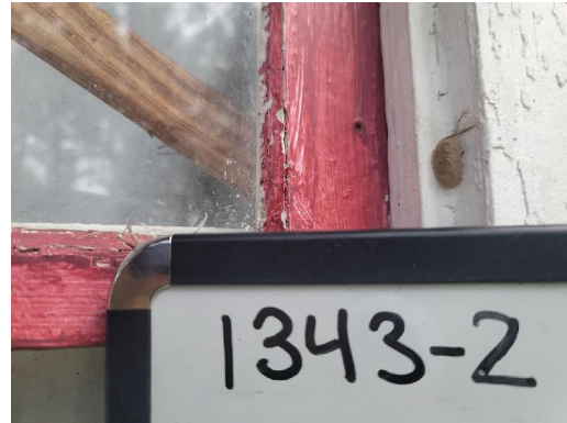
1343-2 Glazing Typical Exterior Windows
